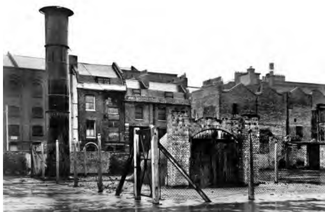
One of 9 entrances to the Southwark deep shelter in Marlborough Yard
